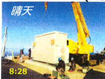
No.3PCS吊り上げ
